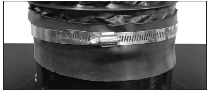
6. Secure the elastic sealing ring and hose with hose clamp
